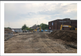
24th May - Reduced dig of metalled road surfaces
