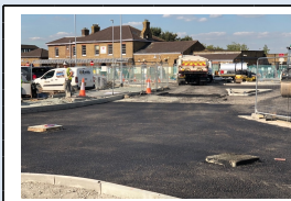
13th September - Asphalt base course being laid in St. Michael's Road
