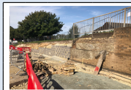
18th September - new blockwork retaining wall being prepared for facing brickwork
