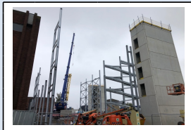
12th September - Continuation of the main steel frame erection
