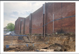
24th May - Reduced dig adjacent to the Forum building
