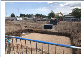
13th June - Excavation of formation for the drainage attenuation crates
