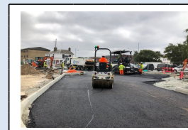
22nd August - Asphalt base & binder courses being laid
