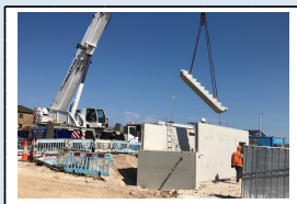
24th July - Construction of the Eastern precast concrete stair core
