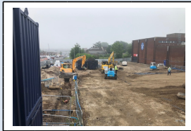
31st May - Formation of the piling mat
