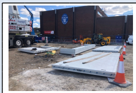
31st July - Precast units stair core units ready to be installed
