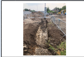
24th May - Excavations to disconnect existing street lighting
