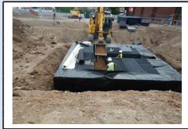
15th June - Installation of the attenuation crates and shingle
