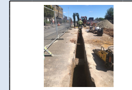
20th June - Clancy Docwra installing new water mains
