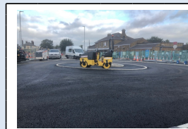
17th September - Asphalt binder course being laid on the new roundabout
