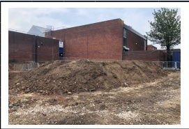
24th May - Stockpiling of excavation material on site
