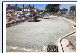
6th August - sub-base being installed in the new taxi rank area
