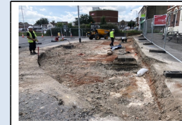
15th June - Excavation of existing road layout
