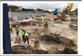
10th July - Formation of the pile cap foundations
