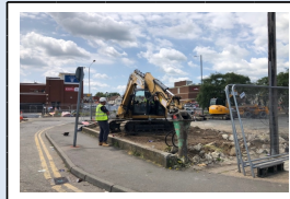
13th June - Site clearance works underway
