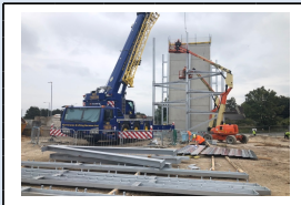
4th September - Erection of the main steel frame in progress
