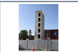
7th August - Eastern Stair Core complete
