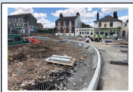
31st July - New kerb line installed for Dover Street
