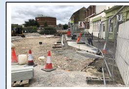
10th July - New kerb line installed in Dover Street
