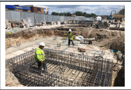
17th July - Steel cages installed for left and stair core foundation
