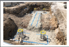
17th July - Some foundations poured throughout the site
