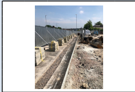
15th May - Site hoarding completed
