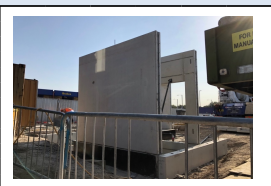
7th August - Assembly of the Western stair/lift core
