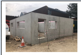
4th September - Assembly of the CCTV/Facilities Room
