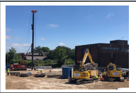
27th June - Piling taking place on site
