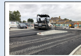
23rd August - Asphalt base & binder courses being laid
