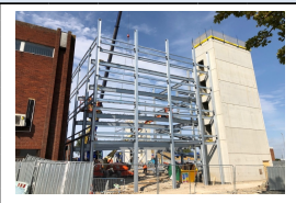
18th September - Erection of the first of the steel floor beams
