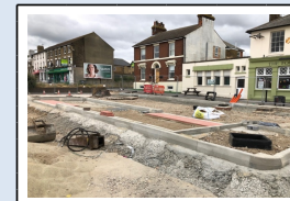
10th July - Installation of tactile paving and traffic light pole sockets
